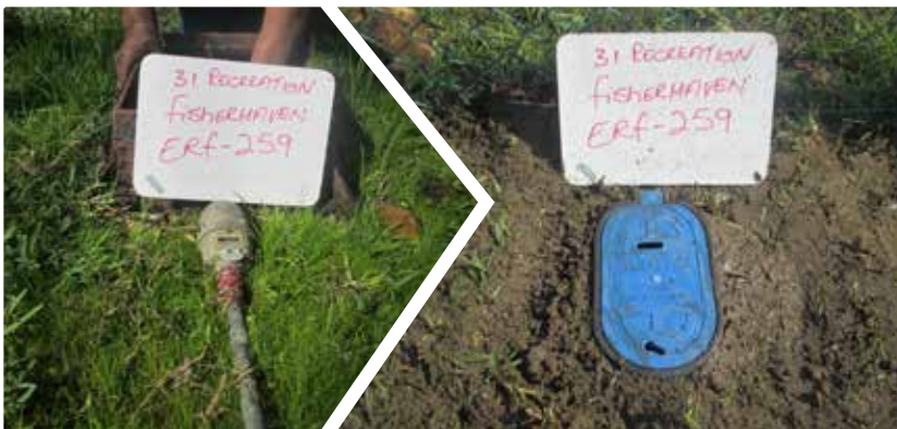
Before and after meter installation by iX Engineers
