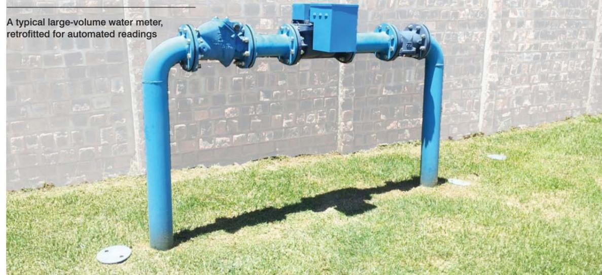
A typical large-volume water meter, retrofitted for automated readings
